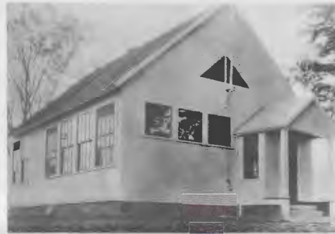
Center School remodeled in the '40s
