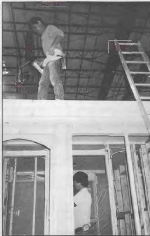
Carpenters working on a house-to-be inside the plant
