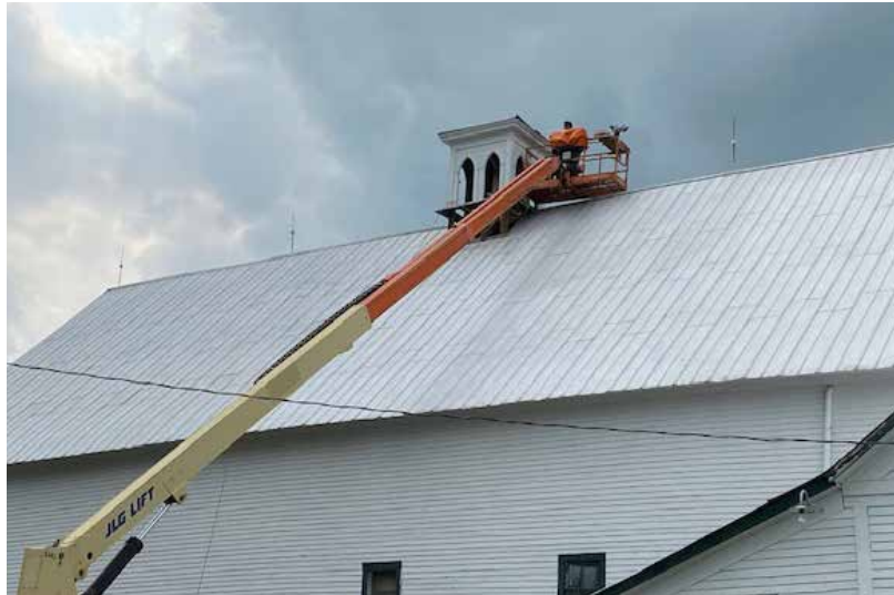
Colin Blackwell installing the new cupola.
